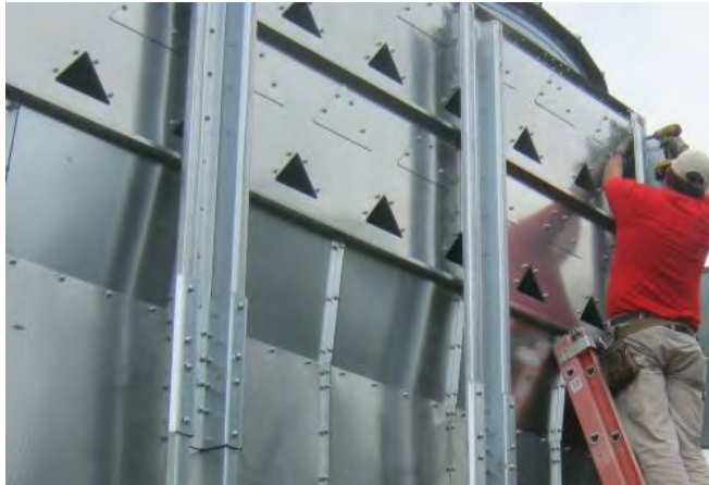
Image 2-3 – Tightening stiffener bolts
