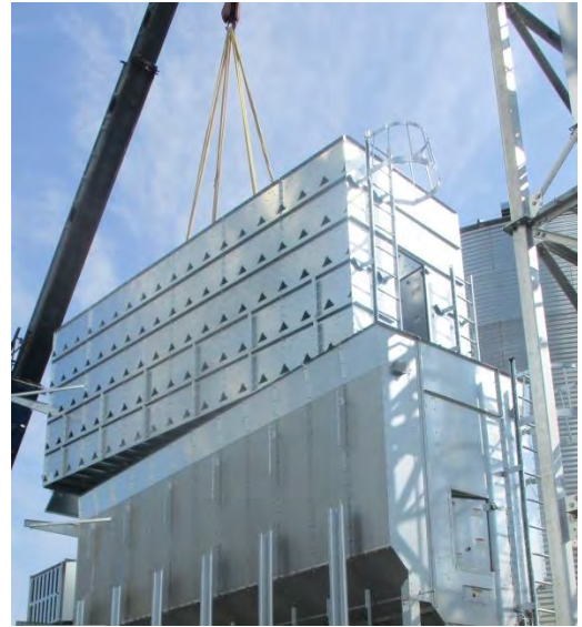
Image 2-4 – Lowering mixing tiers onto cooling section
