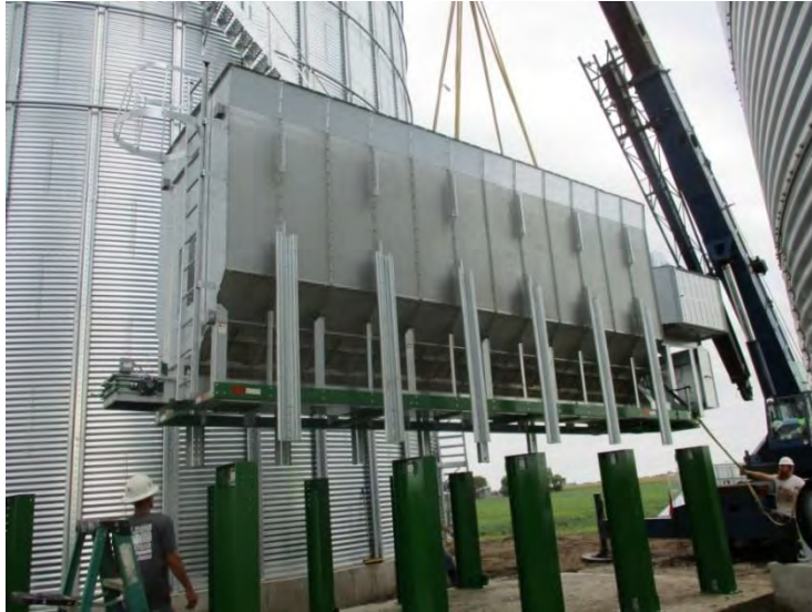
Image 2-1 – Lifting dryer base into position over foundation
