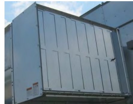
Image 3-4 – Adjustable louvers (shown fully closed)
