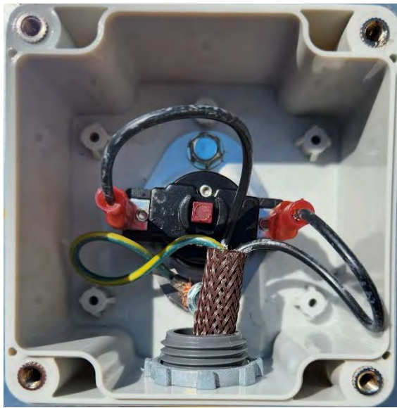
Image 4-16 – Heater housing high-limit switch
