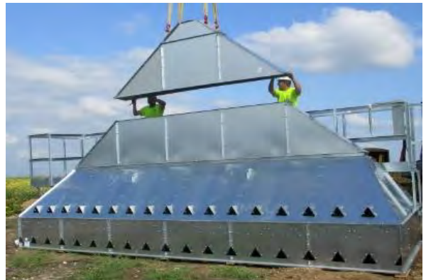
Image 2-5 – Attaching peak section to roof module
