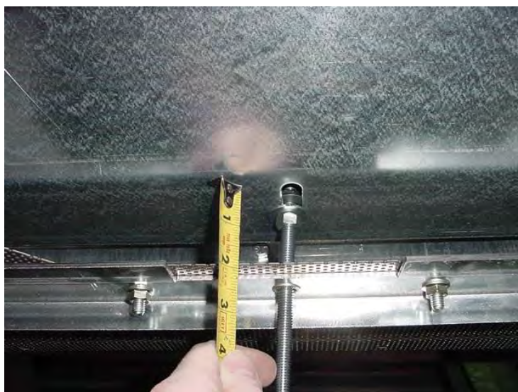
Image 4-33 – Flow gate adjustment
