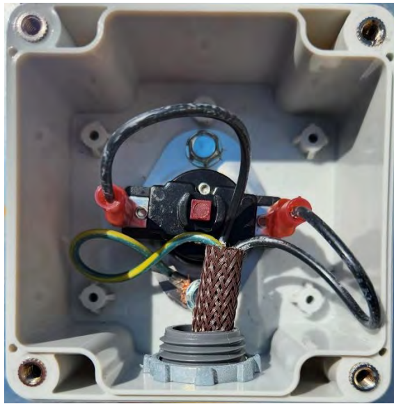
Image 4-14 – Heater housing high-limit switch
