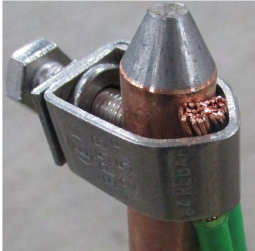
Image 2-3 – Wires clamped to ground rod
