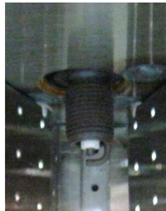
Image 4-31 – Spark plug (shown on H burner)
