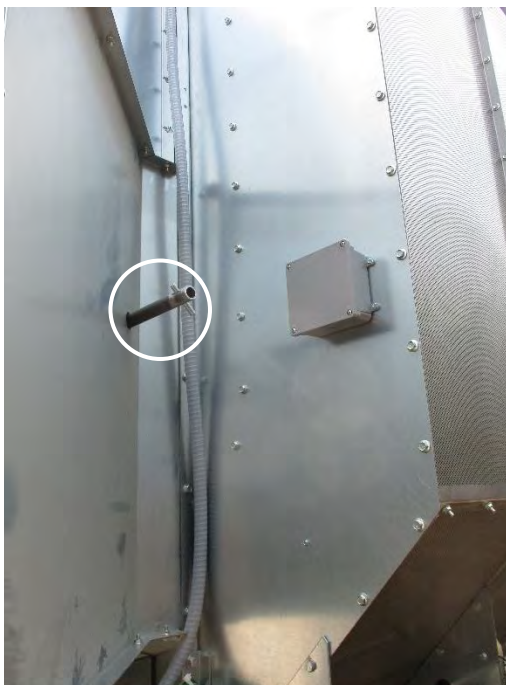
Image 35 – Vacuum-cool door opener handle attachment location
