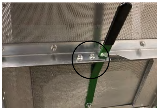
Image 24 – Outer grain column cleanout door
