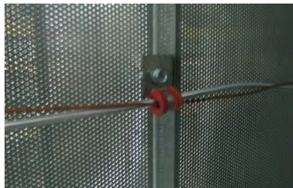
Image 4-40 – RTD temperature sensor wire
