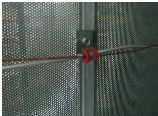
Image 16 – Plenum RTD (silver) and over-temp capillary (copper)
