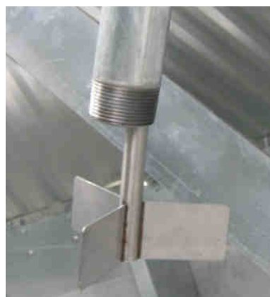
Images 4-2, 4-3 – Upper rotary fill switch, fill sensor
