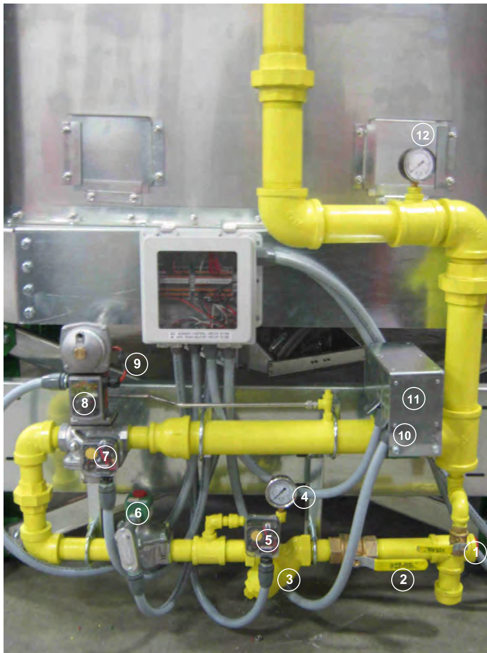
Image 7 – Natural gas-fueled modular tower dryer pipe train components
