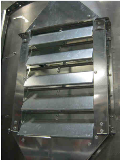
Image 23 – Louvers on door
