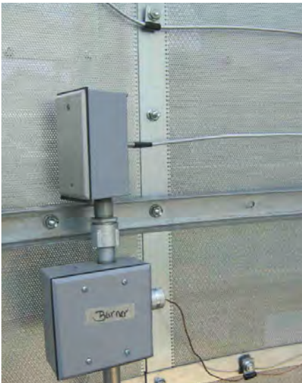
Image 28 – Plenum RTD, capillary box
