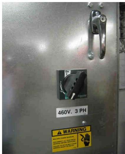
Image 2-2 – Main Disconnect switch in "Off" position
