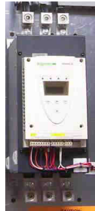
SOFT START CONTROL WIRING
