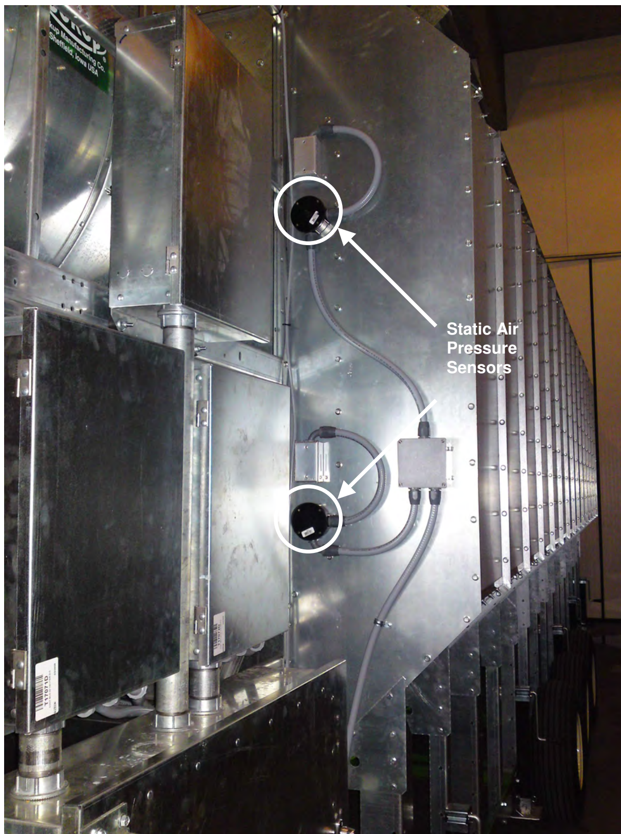
Figure 1.9d: Static Air Pressure Sensors Installed on Dryer (Located in same box as Plenum Over-Temp Sensor.)
