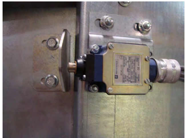
Figure 1.5b: Rear Door Switch
