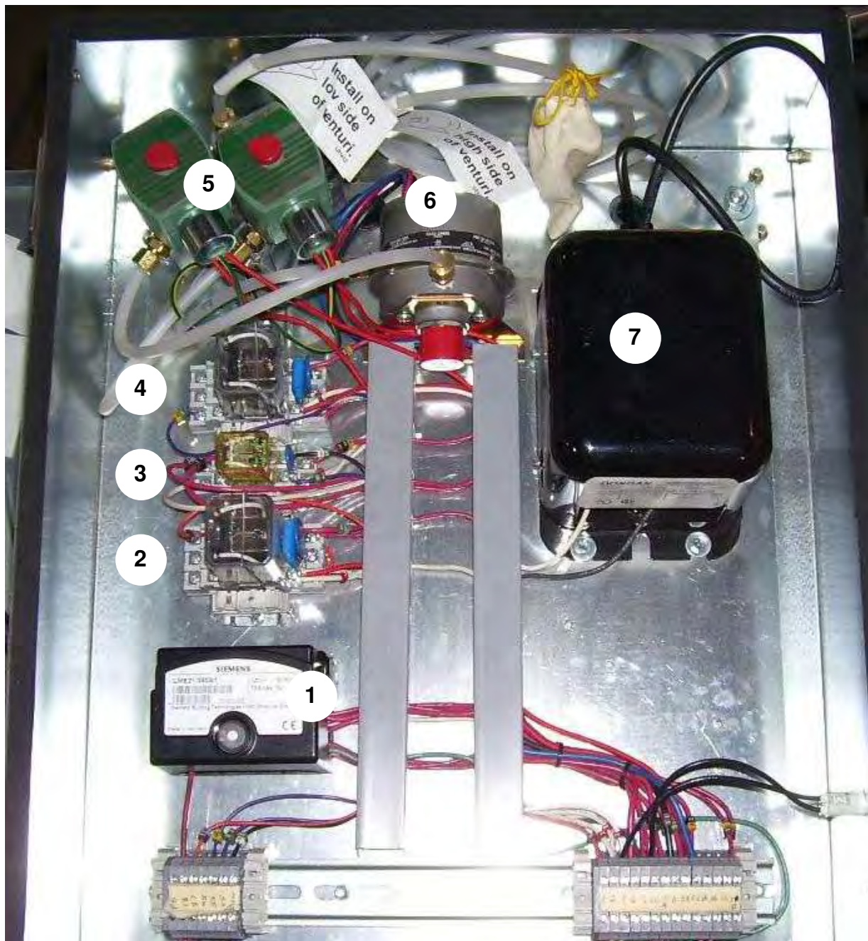
Burner Control Panel for a 38"/44" heater. Components for a 28" heater are the same minus the LDU11 flame proving unit.
