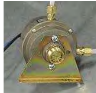
Figure 1.9c: Differential Air Switch (Located in Heater Box)
