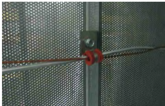
Image 4-30 – RTD Temp sensor wire
