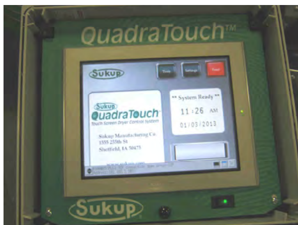
Image 44 – Main power switch on
