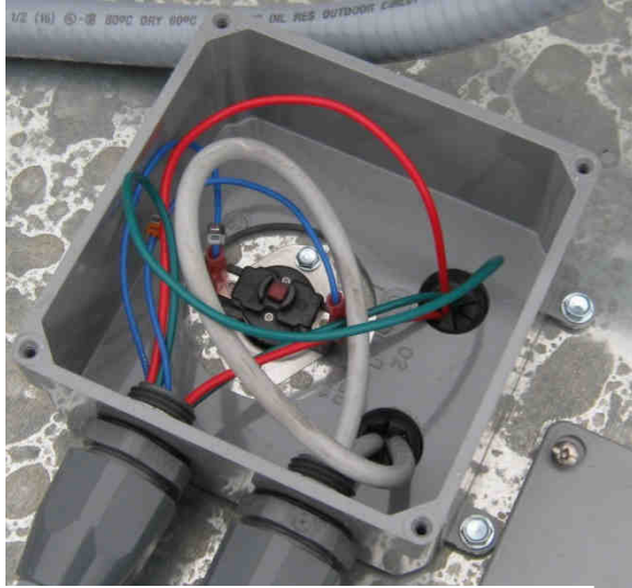
Image 4-9 – Heater housing high-limit switch
