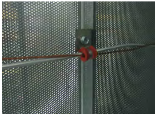
Image 12 – Plenum RTD and over-temp capillary
