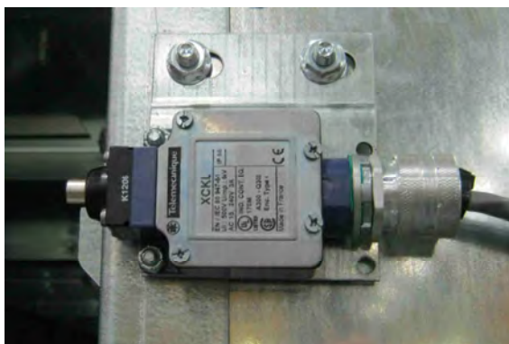
Image 5-10 – Rear door interlock switch
