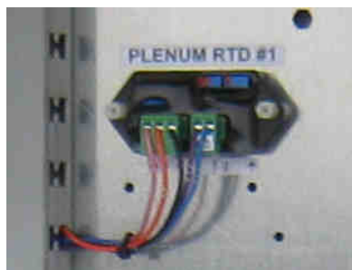
Image 4-11 – Plenum temperature sensor (RTD) transmitter in power box. See Item 16 in Image 6 of Component Identification section.
