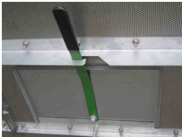
Image 4-34 – Grain column outside cleanout door handle
