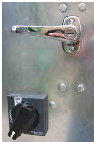
Image 21 – Latch and switch in “Off” position
