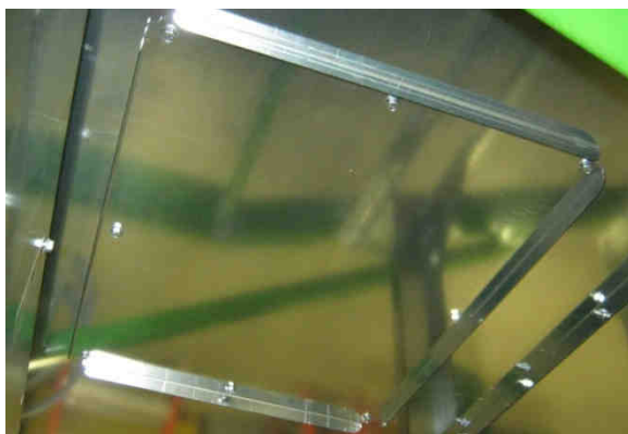
Image 4-36 – Vacuum-cool duct cleanout door
