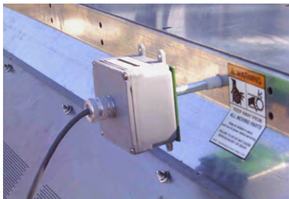
Image 26 – Paddle switch box in operating position
