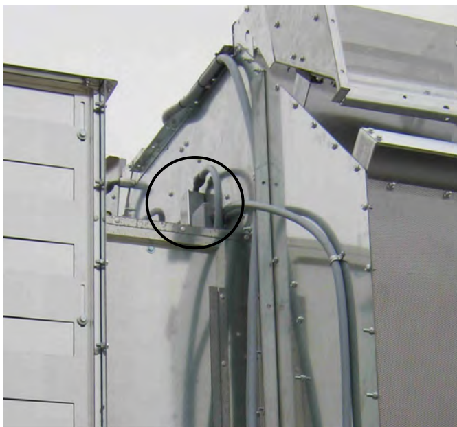
Image 5-24 – Plenum temperature sensor
