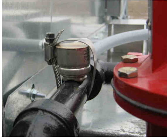
Image 4-6 – Vaporizer over-temp switch
