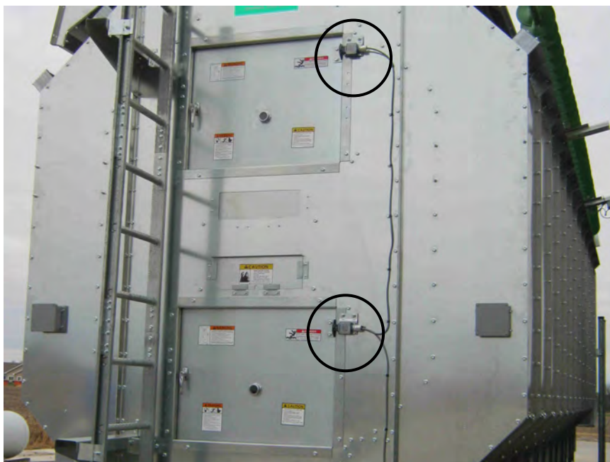
Image 5-11 – Rear door interlock switches
