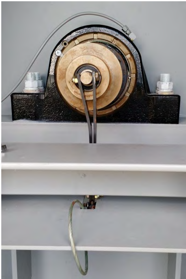
Image 3-8 – Backspin preventer installed
