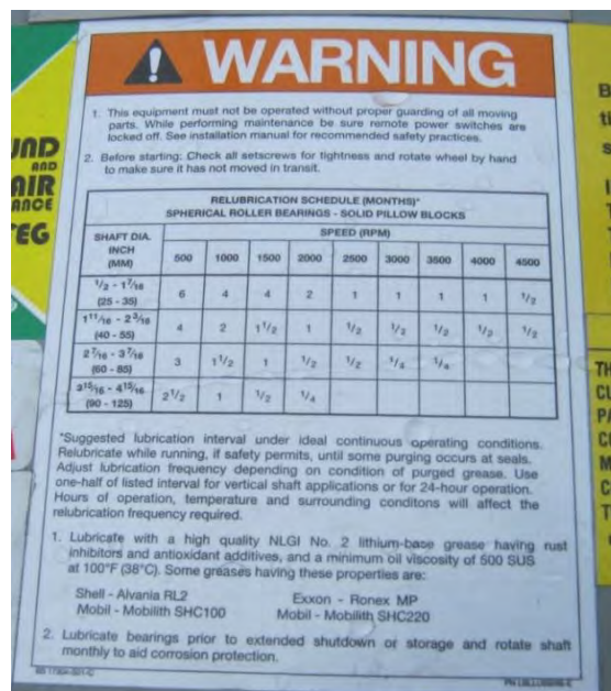
Image 3-2 – Twin City Fan & Blower lubrication sticker
