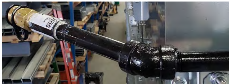
Image 2-11 – Extending relief pipe past side of dryer
