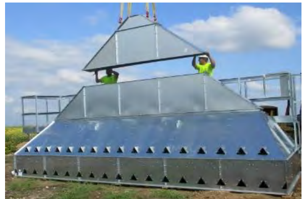
Image 2-5 – Attaching peak section to roof module
