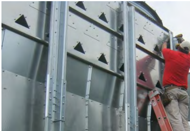
Image 2-3 – Tightening stiffener bolts
