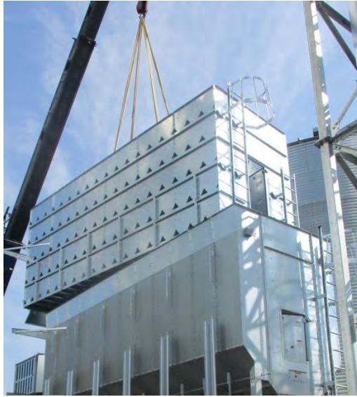
Image 2-4 – Lowering mixing tiers onto cooling section
