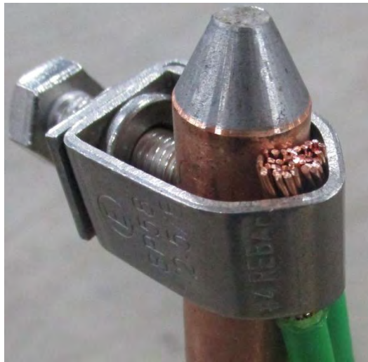
Image 2-21 – Wires clamped to ground rod
