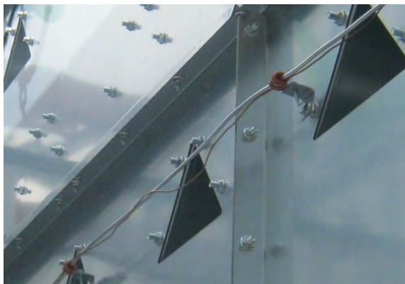
Image 4-44— RTD temperature sensor tube (aluminum)
