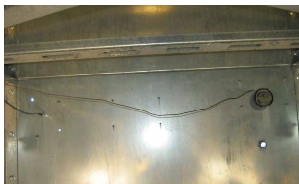
Image 13 – Plenum RTD (thermometer) tube & static air pressure switch screen
