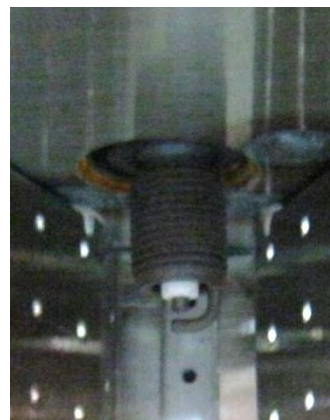
Image 4-31 – Spark plug (shown on H burner)
