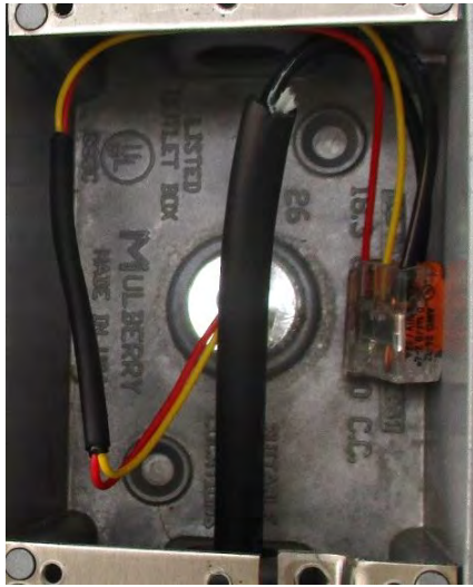
Image 4-15 – Plenum temperature sensor RTD
