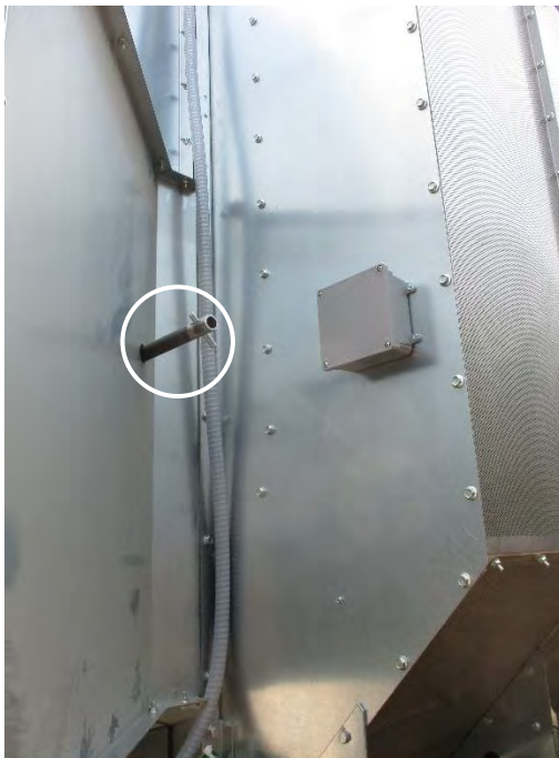
Image 35 – Vacuum-cool door opener handle attachment location
