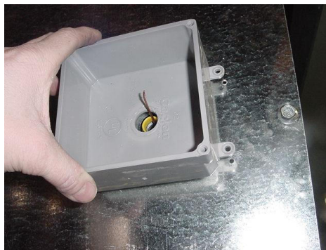
Photo 1.1: Removal of rear column over temperature box
