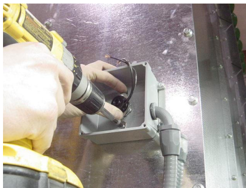
Photo 1.4: Installation of the high limit switch to the right rear of the dryer
