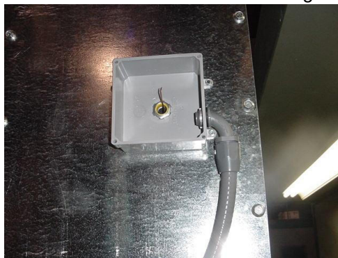
Photo 1.2: Reinstallation of right rear column over temperature junction box after attaching supplied conduit
