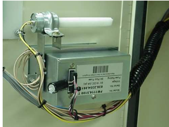
Figure 2.2b: Paper Roller Installed
