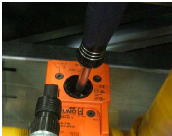
Image 7 – Setting valve to 0% open
